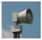
ThorGuard Lightening Prediction system on the roof of the Recreation Building will sound a long (15 seconds) horn when lightening conditions exist. A strobe light will also activate. Seek cover immediately. Three short (five seconds each) horns will sound when the area is clear of the lightening threat.
